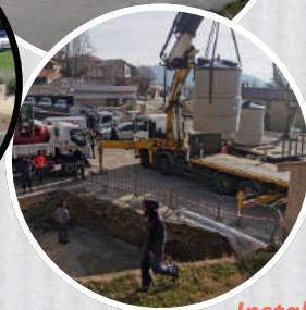
Installation des conteneurs semi-enterrés
